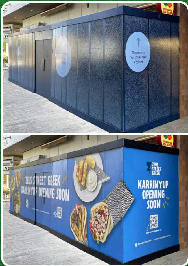
Same installation with Gboard wrapped with Pform PP PVC-free SAV and Protect-PRO Laminate PVC-free.
